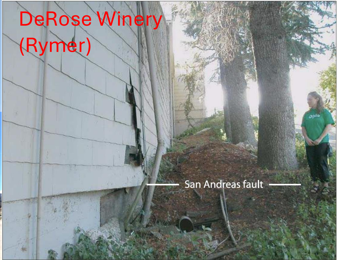
Figure 13. Northwest wall of DeRose Winery showing evidence of incremental creep (fault slip) along the San Andreas fault. View is to the southwest; photograph taken November 2005.
