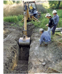
Trenching across the Hayward Fault in Fremont
